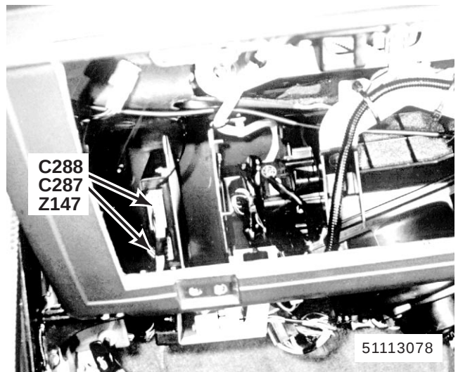
78. behind LH side of fascia Z147 Window Lift ECU C287 (10-W) C288 (8-W)
